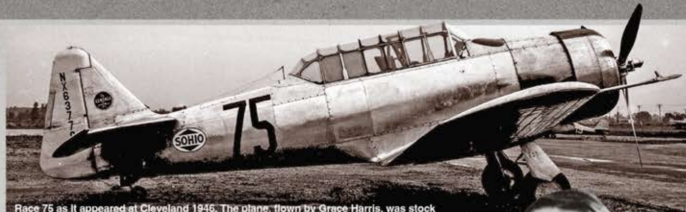
Race 75 as it appeared at Cleveland 1946. The plane, flown by Grace Harris, was stock except for the addition of a three-blade propeller.
