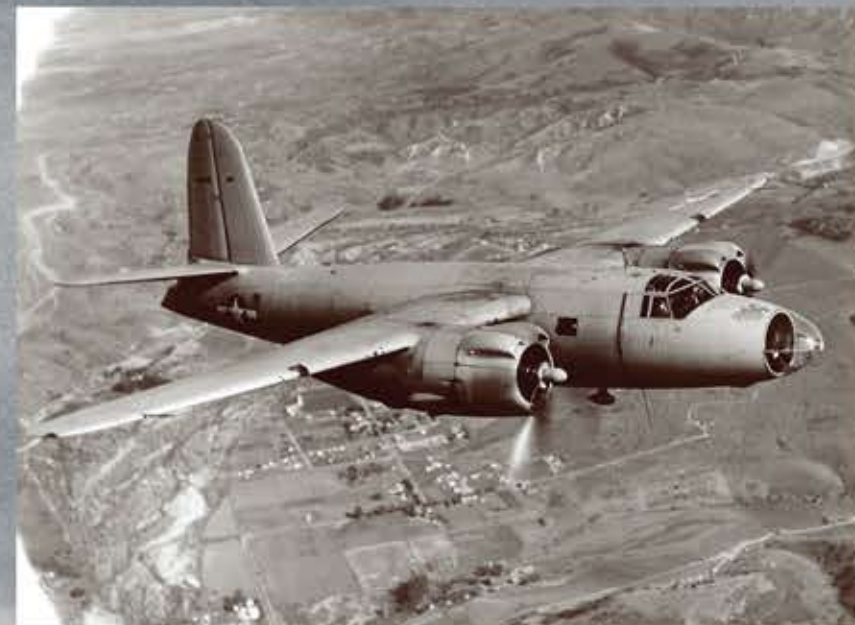
Its overall yellow paint a bit faded, JM-1 BuNo 66783 was photographed in 1945. Note the completely empty nose area and where the rear fuselage turret was covered over. (William T. Larkins)
