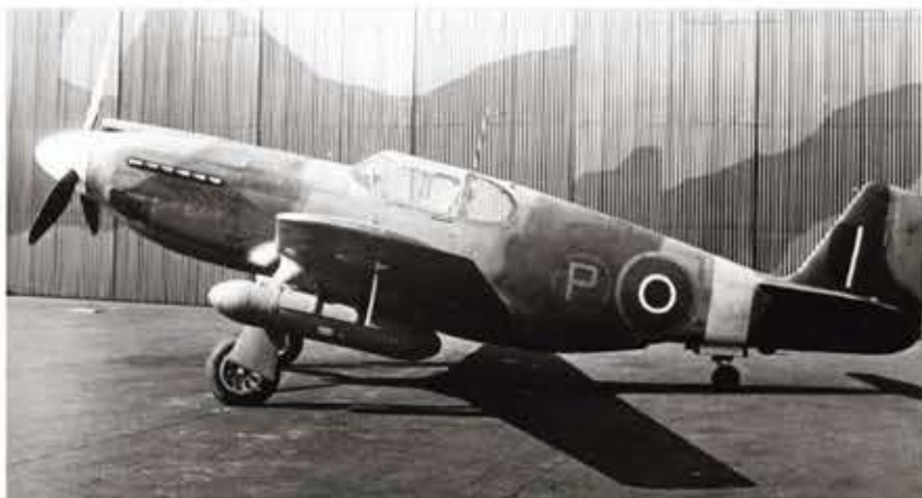
Mustang Mk. I AM106 at Boscombe Down testing an underwing stores pod. Note that all armament has been removed.
