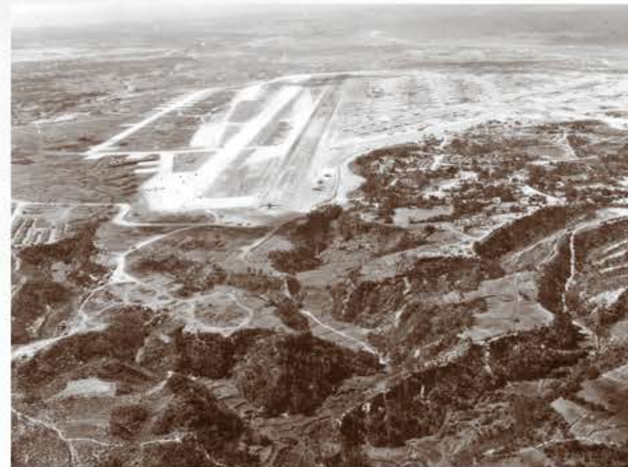
Yontan was a vital airfield and immediately after capture, Americans went to work to expand and improve the facility.
