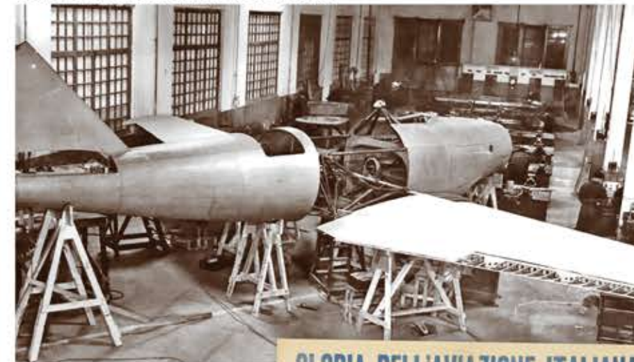
This view of the prototype under construction shows the large engine bay and the allerons that would receive a fabric covering.
