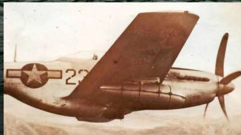
Mustang carrying a prototype Josephine tank.
